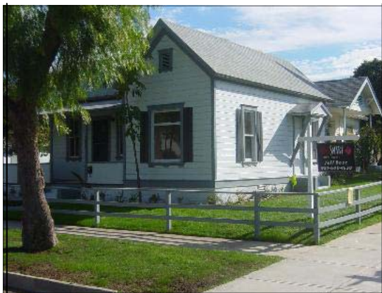
The Brumbaugh House as it looked when named to Corona's Historic Landmark List.
