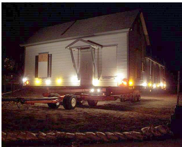
The house atop transport dollies, illuminated and ready to be moved off the 300 block of West Seventh Street in the dark of night, onto Belle for its journey to the rear of 1052 E. Grand Blvd, via Sixth Street, Main Street, Grand Boulevard and Howard Street.
