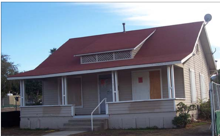
312 West Seventh Street It would be a shame for this to end up in a landfill!!
