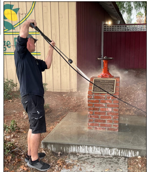
Pressure washing the base of marker No. 12 at Corona Foothill Lemon Ranch headquarters at 510 Foothill Parkway
