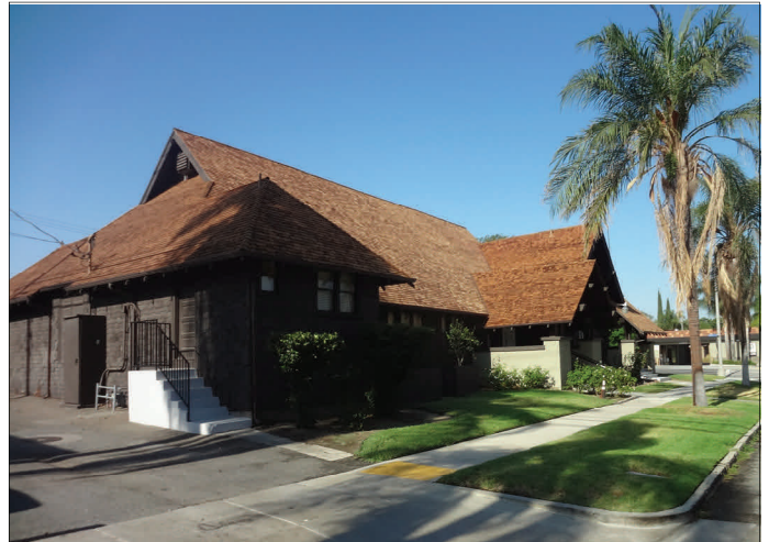
Completed north facing gabled main roof, gabled north portico, northeast hipped roof and east side/end of clubhouse.
