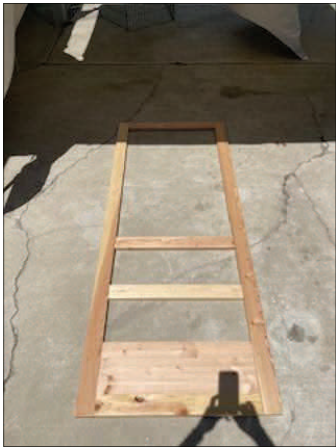
Basic wooden door frame with a header, two cross pieces and a footer.
