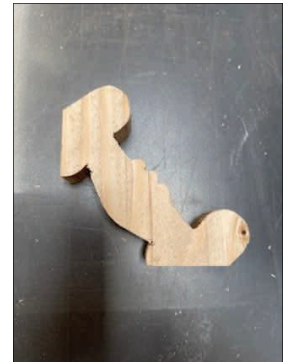
A piece of scroll work to be placed in the corners of the screened opening in the door to provide a Victorian “gingerbread” detail.
